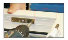
Position the striker plate behind the bead groove on the outer frame 45mm from the corner and screw into position.
