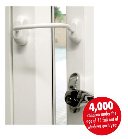
A small yet very effective and extremely affordable solution is the UAP window restrictor. The window restrictor has a 20cm long cable, which when installed correctly will limit the opening of the window to under 100mm. Not only will this prevent children from being able to fit through the gap, but it also allows enough air to circulate around a room.
